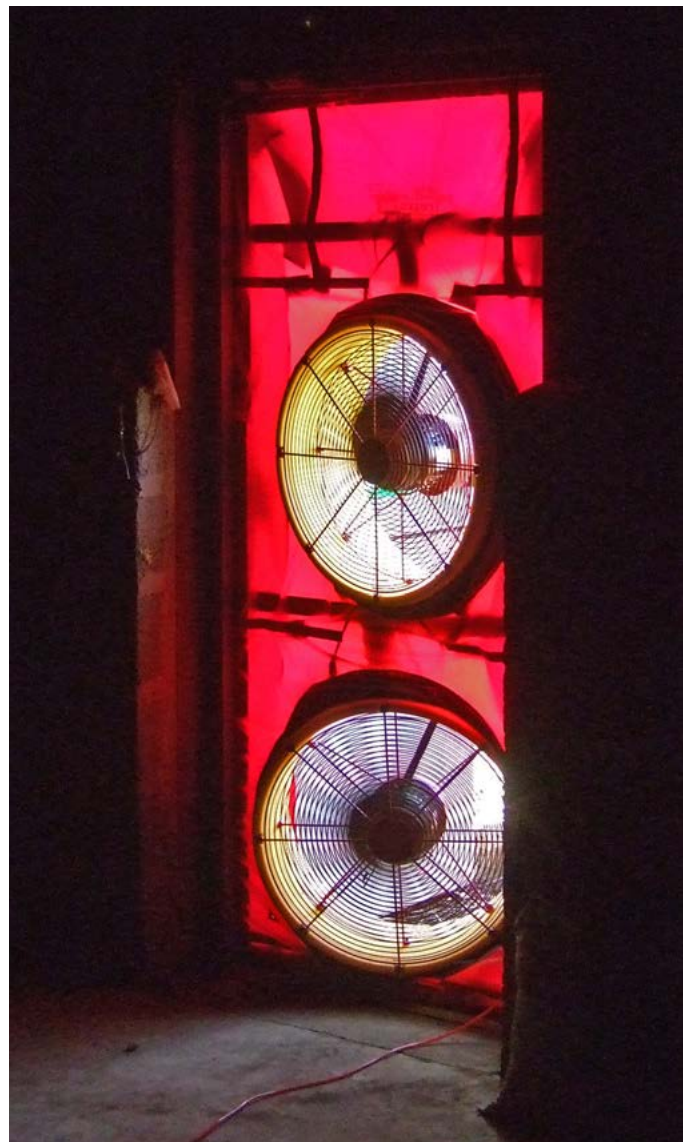
Figure 3. Air leakage assessed by forced introduction of air and monitoring pressure change
