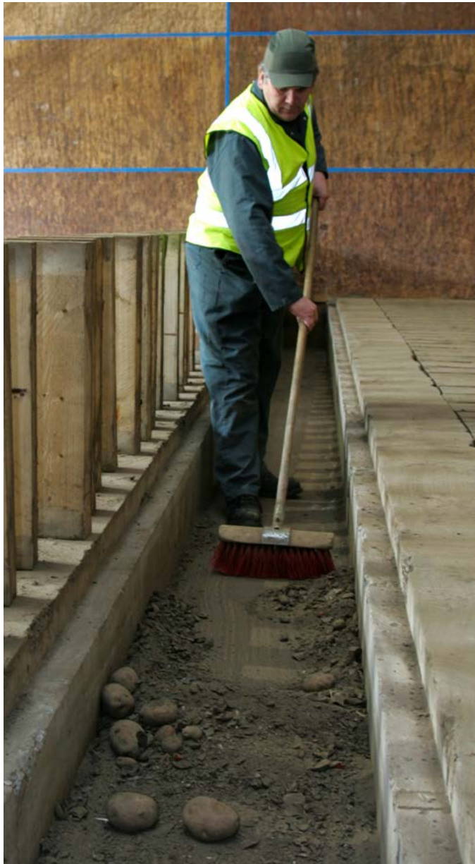
Figure 8. Remove all debris before loading
