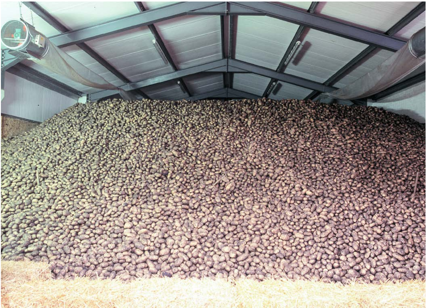
Figure 19. Roof space heating in a bulk store
