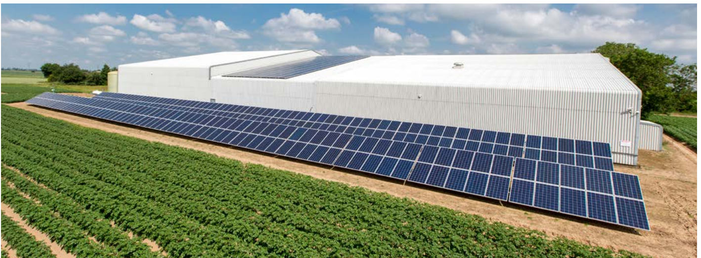
Figure 26. Refrigerated potato stores can make good use of solar energy in summer months
