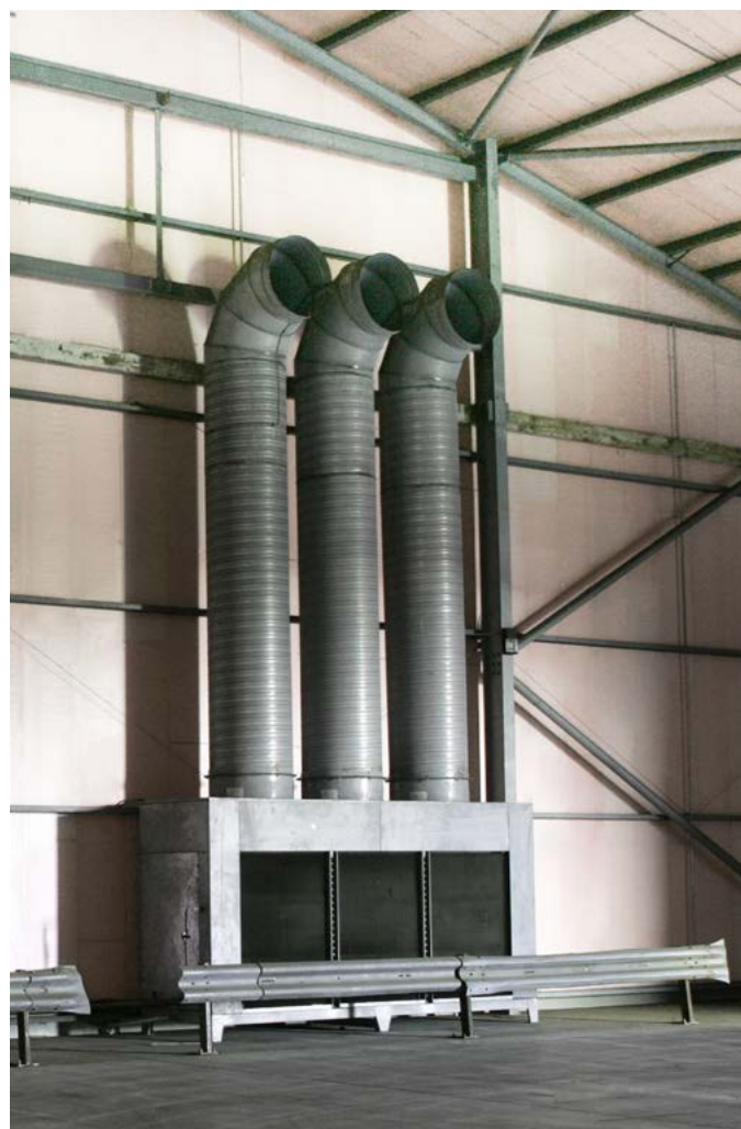
Figure 20. Floor-mounted fridge unit typical of older installations
